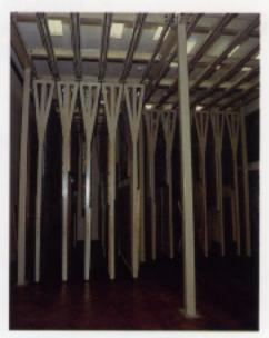
A Tuff-Track truck was then mounted to each end of the header bar and aligned with the 18" on-center parallel track runs, forming a mini bridge crane-type carrier at either panel end. To eliminate weld or fire damage to the valuable parquet floor, mechanical fasteners were used exclusively throughout the system.
